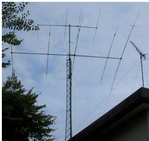
Half of one of the directors of Shi's four element 10 metre yagi is missing.
